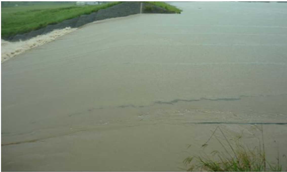
An emergency spillway engages on a dam complicating downstream flood impact
